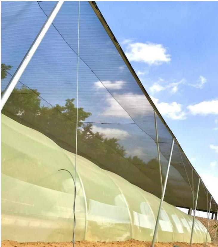
**Figure 2** – Tunnel greenhouse of the AWESOME lab scale facility with a shading cloth for protection against radiation and heat.
