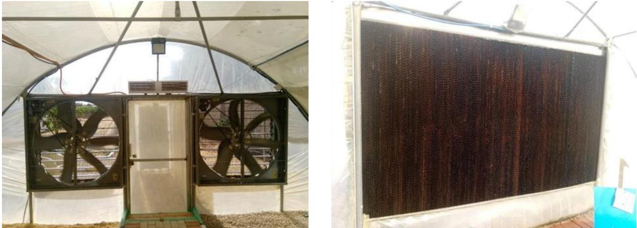
**Figure 1** – Fans (left) and cooling pad (right) of the convective cooling system at the head sites of the AWESOME lab-scale greenhouse
